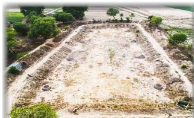
Newly constructed pond for water recharge in MIL-2 unit of Hapur
